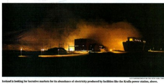
Iceland is looking for lucrative markets for its abundance of electricity produced by facilities like the Krafla power station, above.
